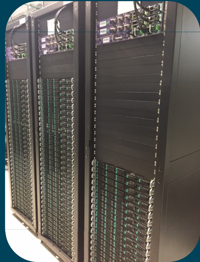
Picture of Validation Racks with 500 nodes at GDC Intel Site
